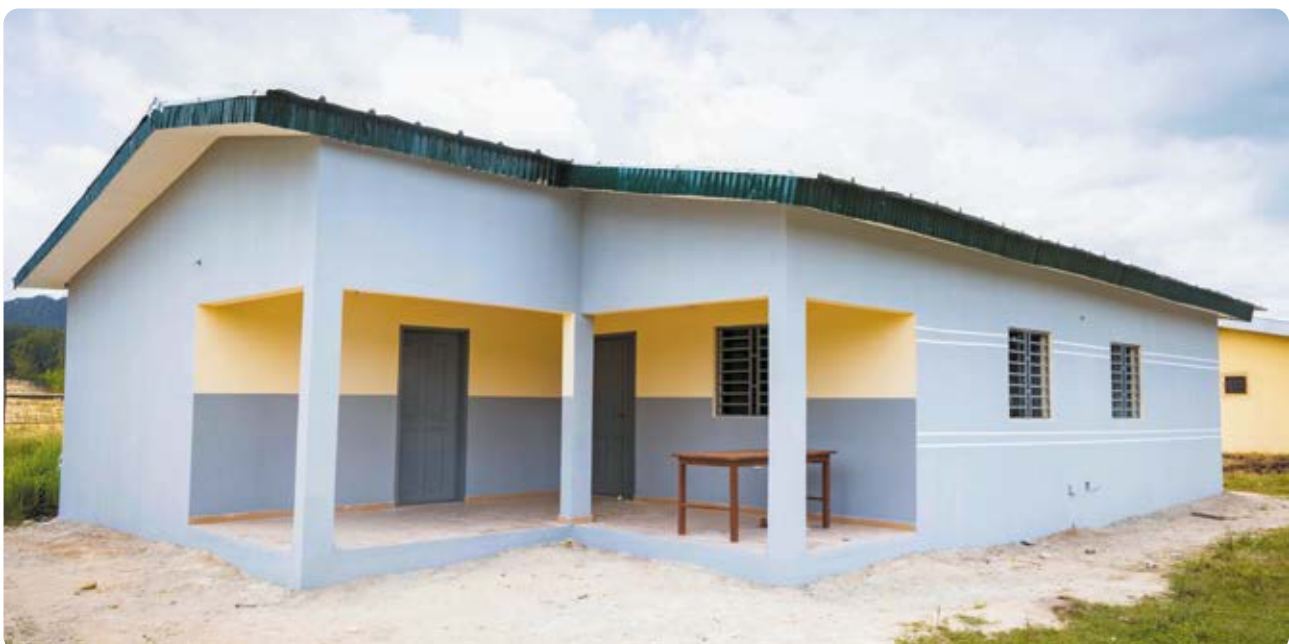
Building of a house for teachers by EPC Côte d'Ivoire
