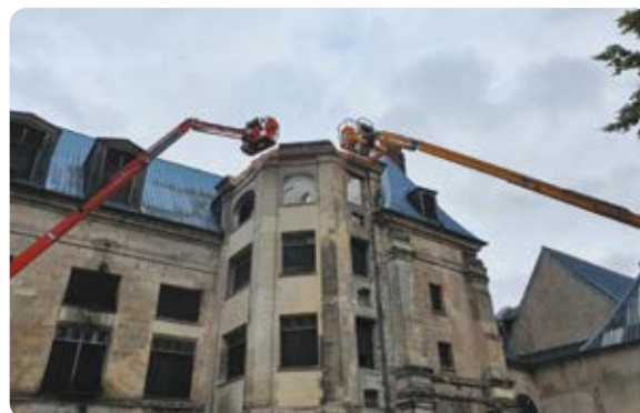
Remediation and demolition works at the Villers-Cotterêts site, France
