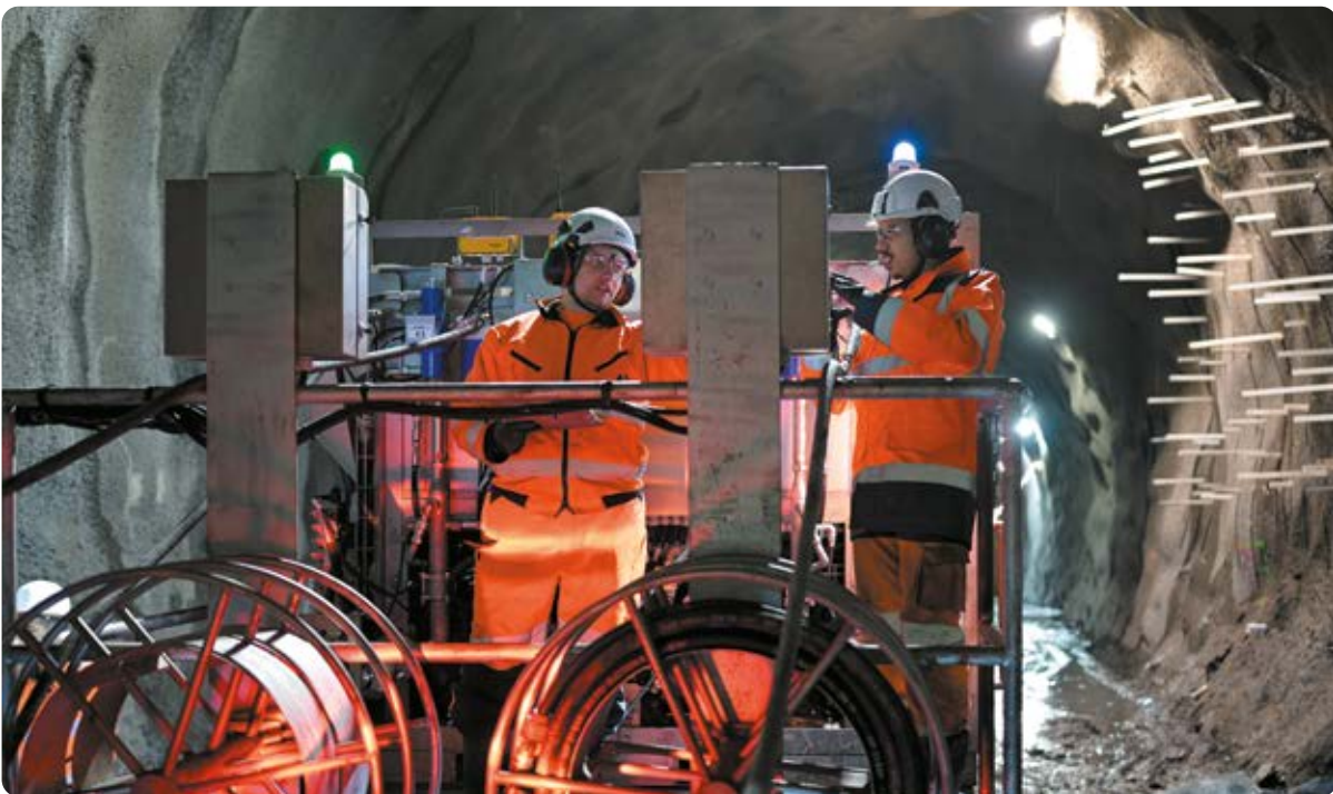
TELT construction site, France
