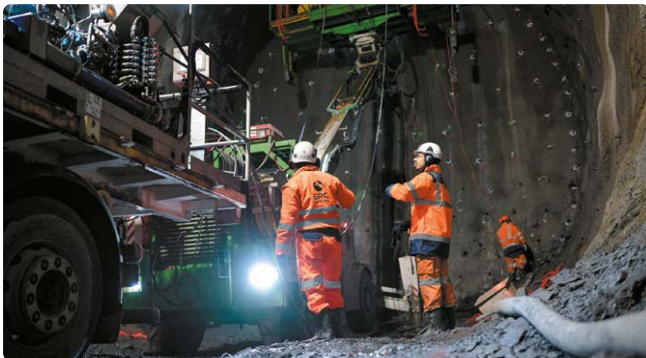
Operators on the TELT construction site, France
