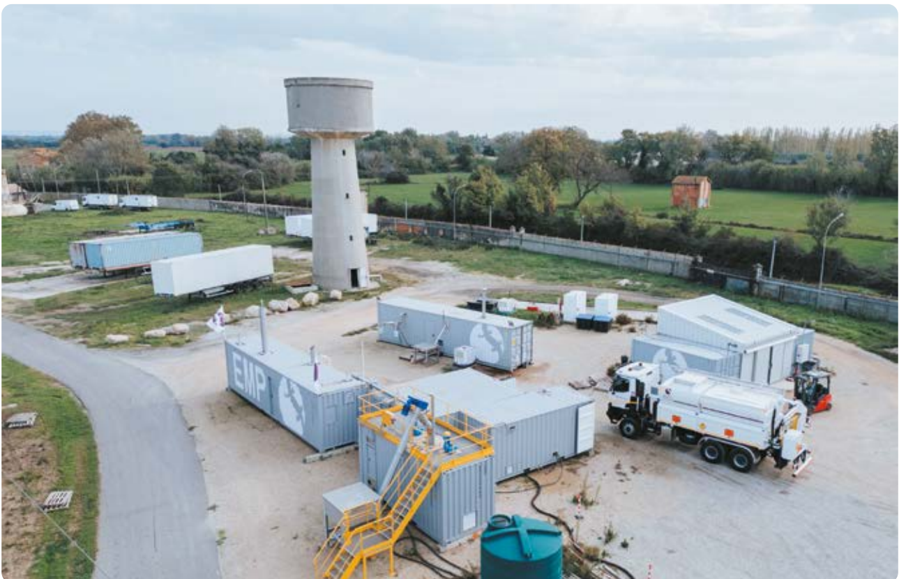
EMP (Euro Modular Plant) on EPC 2i site, France
