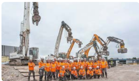
EPC Demosten worksite, France
