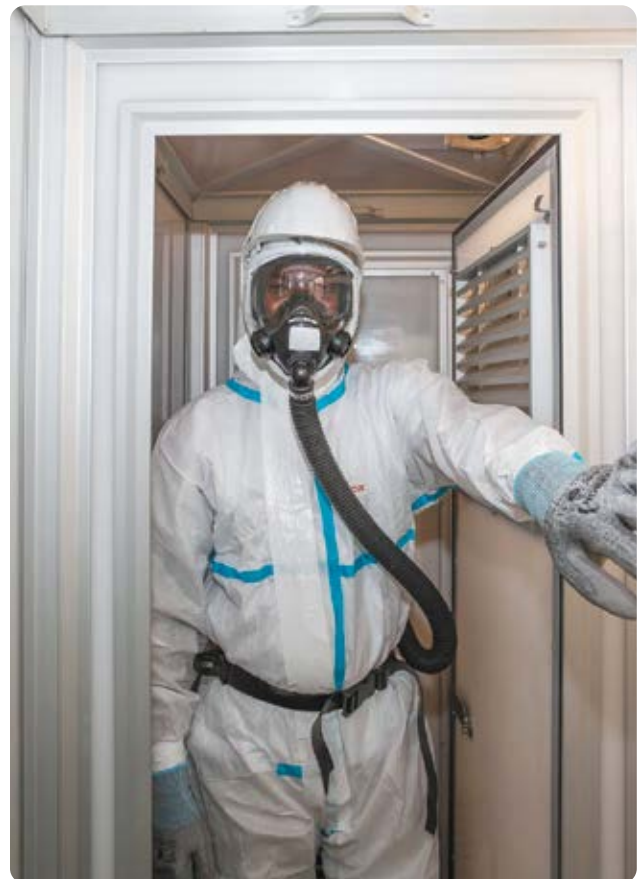
Asbestos removal operator, EPC Demosten, France
