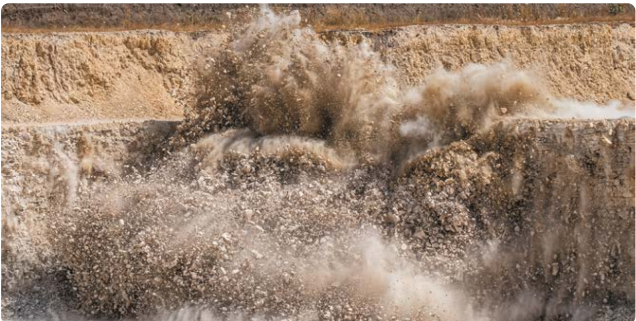
Blasting operation in Senegal
