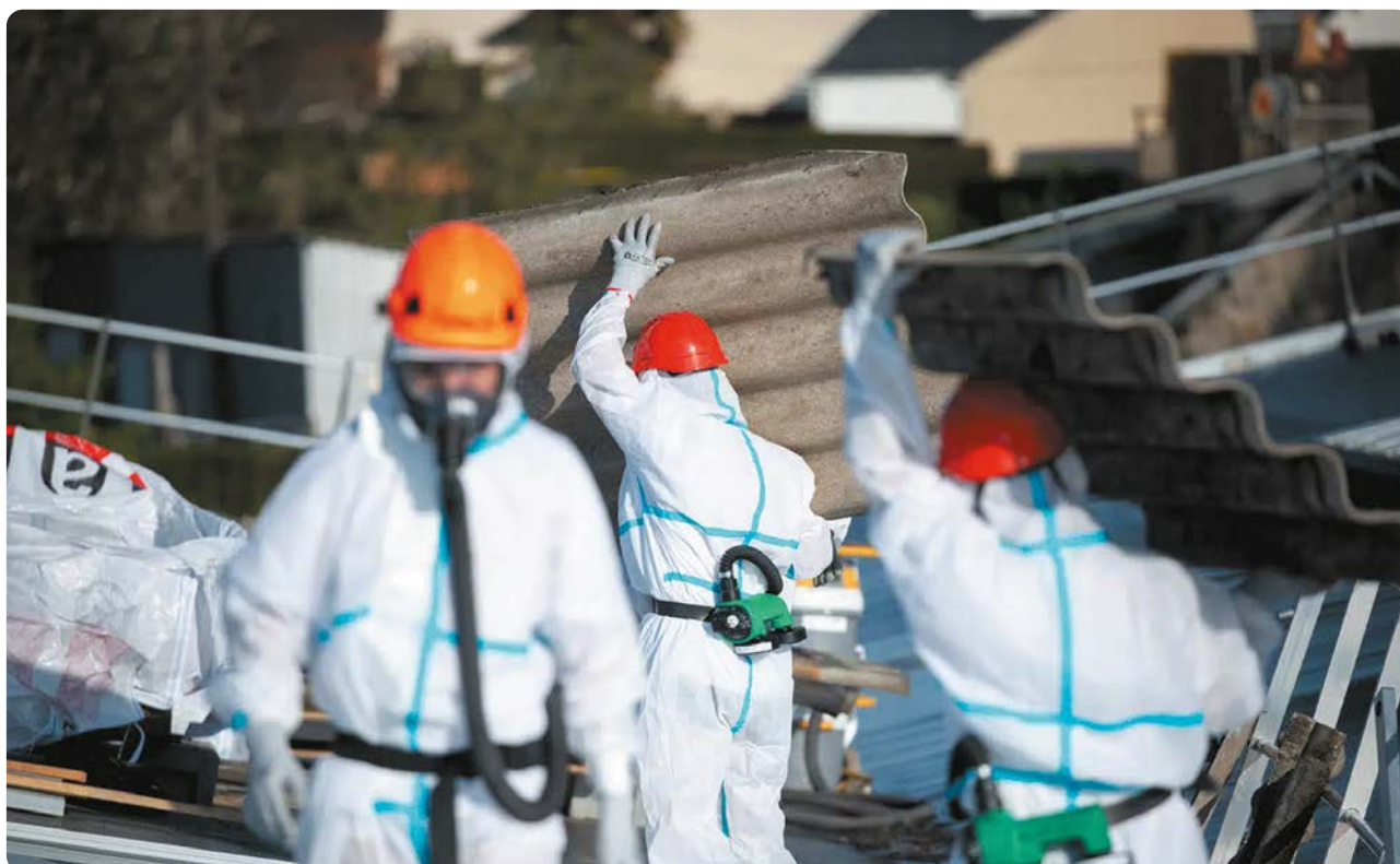
Asbestos removal from roofs and suspended ceilings on an industrial site
